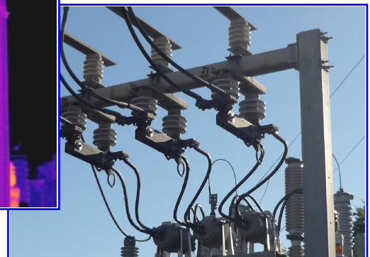
Bad Connection at Switch Shows as Thermal Anomaly
