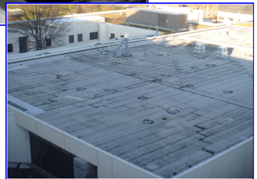
Lighter Color is Thermal Anomaly Indicating Area of Wet Insulation
